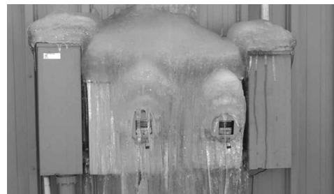
Electric meters covered with ice can lead to damage and outages.
