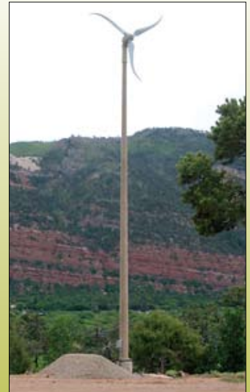
Located in La Plata County, each of these approximately 2.5 kW wind turbines are net metered and interconnected to LPEA's grid — an important component of the cooperative's support of local, distributed generation.
