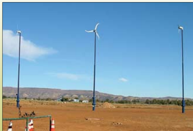
Located in La Plata County, each of these approximately 2.5 kW wind turbines are net metered and interconnected to LPEA's grid — an important component of the cooperative's support of local, distributed generation.
